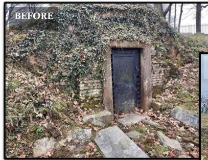
Cleaning of Trabue Vault Frankfort, KY
