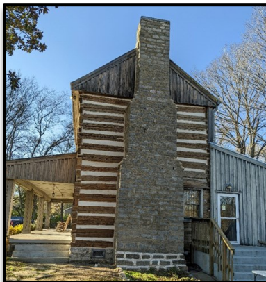
Exterior Restoration of Buchanan Log House Nashville, TN
